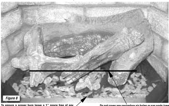
To ensure a proper burn leave a 1" space free of any embers or rockwool directly in front of the air deflector (see Burner Pan Diagram above).
